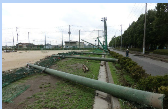
Tornado Damage, Koshigaya, Saitama, 2013
