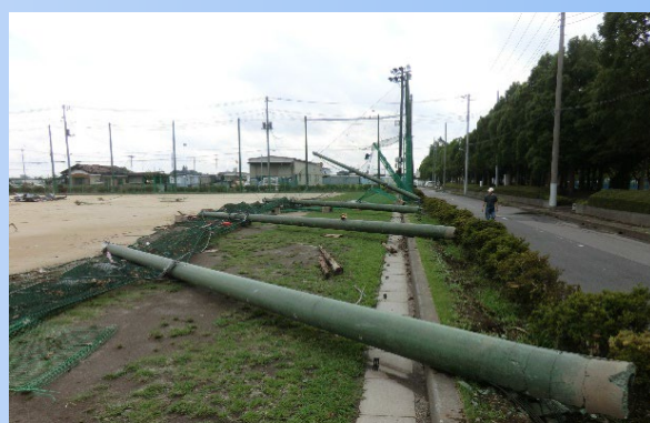
Tornado Damage, Koshigaya, Saitama, 2013
