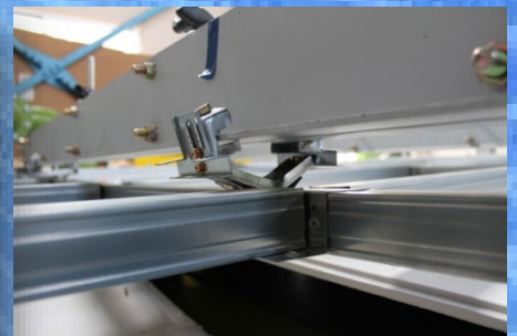
Destruction of ceiling
