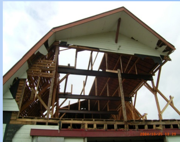
Tornado Damage, Monbetsu, Hokkaido, 2004
